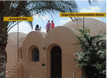
Figure 5: Shows the accommodation rooms in front of the pool
